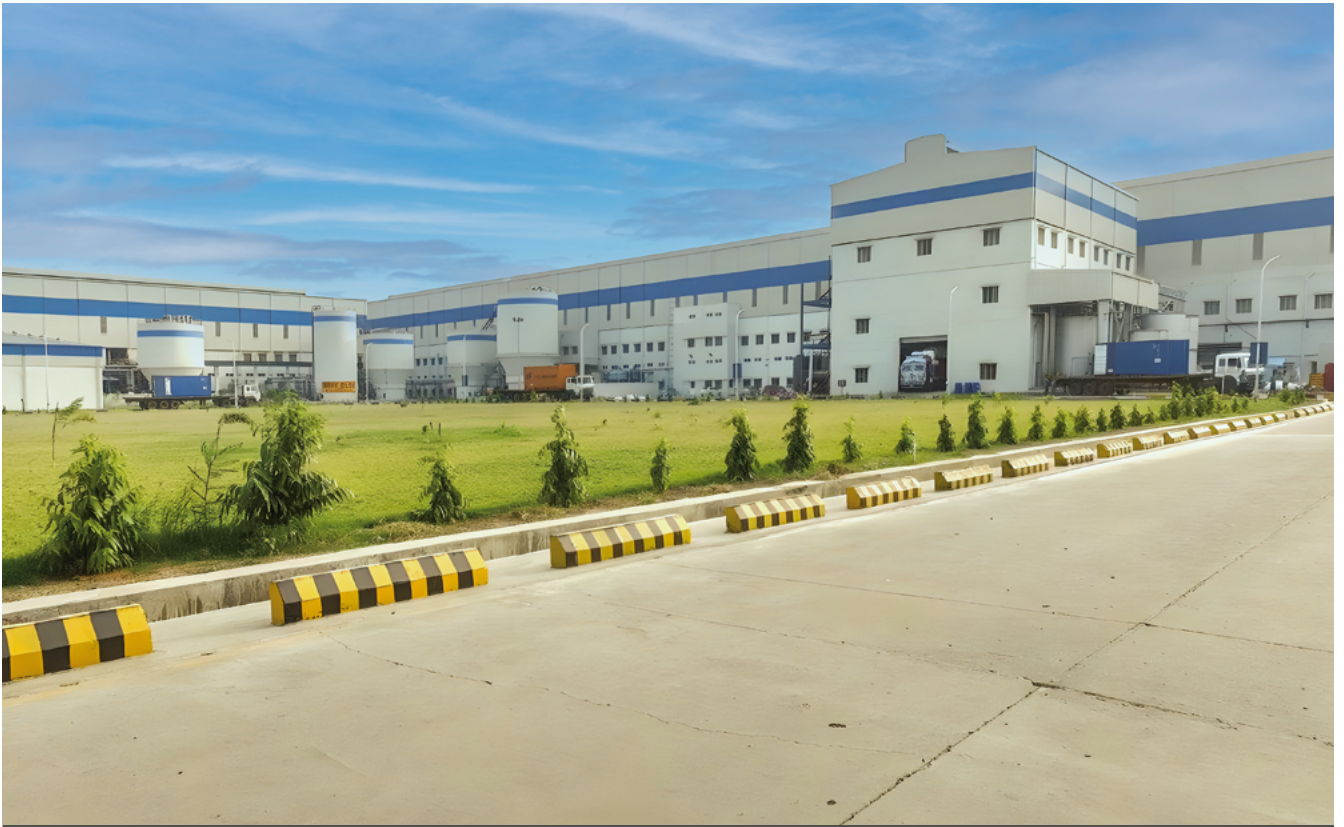
Manufacturing facilities at Balasore, Odisha
